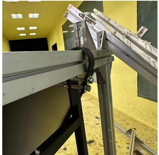
Bracket and bolts fixed
